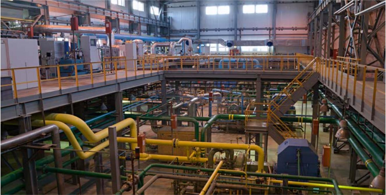
Motors, gas compressors and piping – an ASU machine room has many potential gas leak hazards
