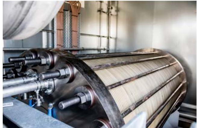
0.5 MW, 200 cubic metres per hour McPhy Hydrogen Electrolyser. Copyright RAG & Karin Lohberger Photography.
