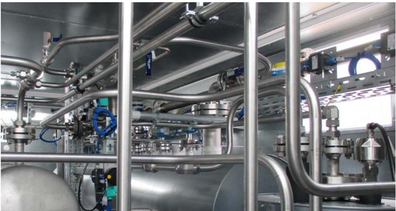
Hydrogen electrolyser installation. Copyright TÜV SÜD.
