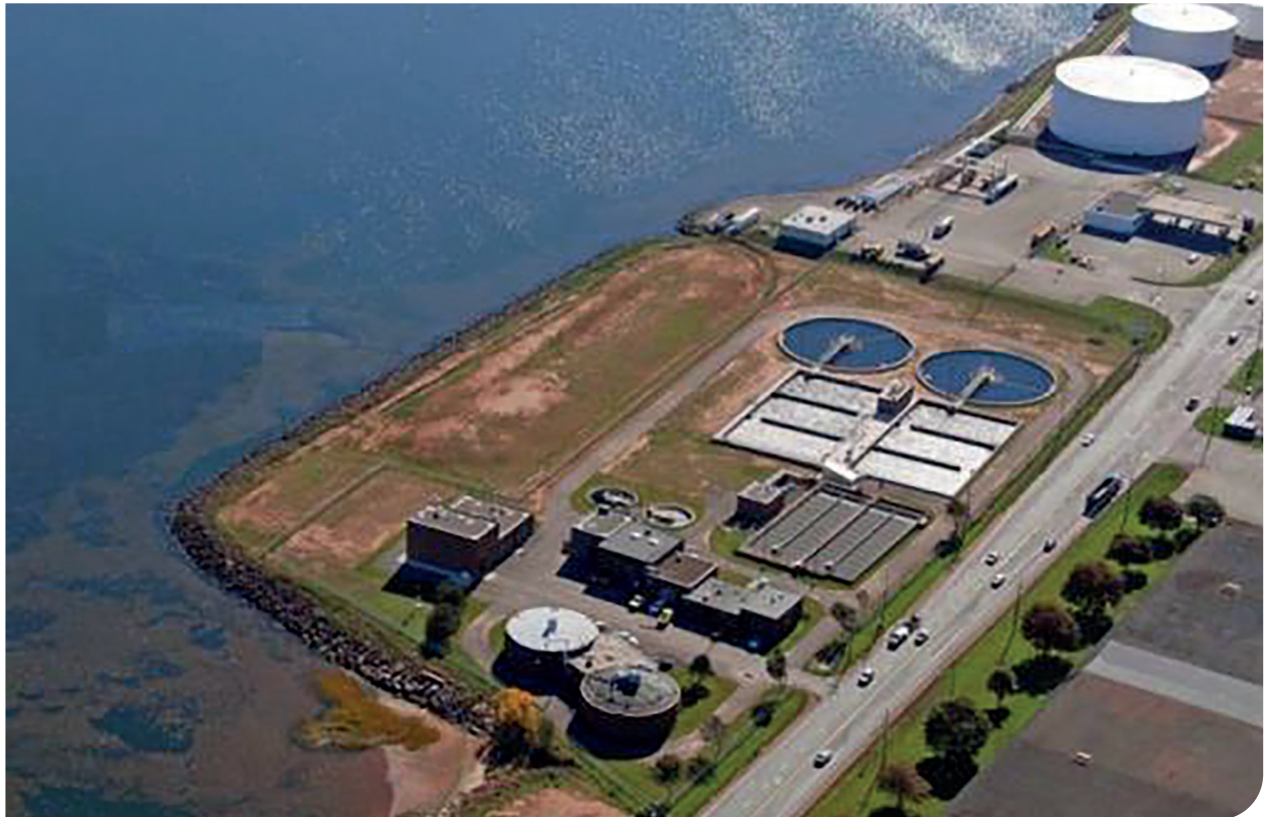
Charlottetown Treatment Plant where they're using SENTRY wastewater sensors upstream to monitor incoming loading and make more accurate aeration adjustments for energy conservation
