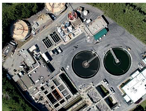
The Sewer Authority Mid-Coastside (SAM) treatment plant where they're using SENTRY wastewater sensors for real-time, early-on influent insight to better manage variable influent from industrial dischargers
