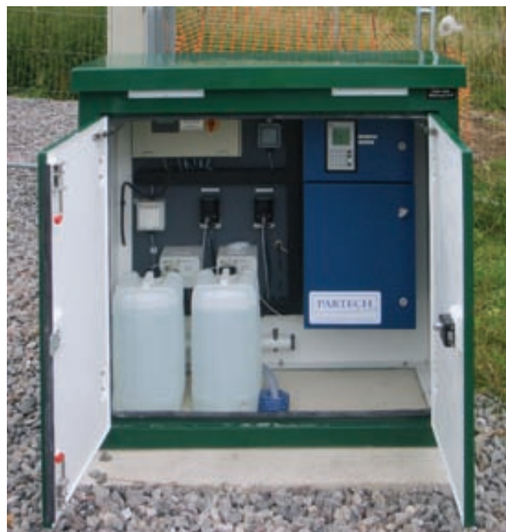
Fig 2: The sampling system is a critical part of the dosing control system, as the analyser requires an optically clear sample to accurately determine the orthophosphate level.
