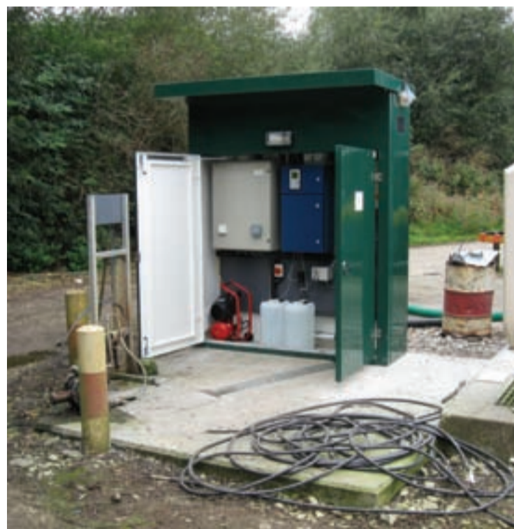
Fig 2: The sampling system is a critical part of the dosing control system, as the analyser requires an optically clear sample to accurately determine the orthophosphate level.
