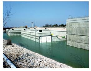
Caissons made of reinforced concrete form the foundation of the flood protection system: KELLER AG für Druckmesstechnik
