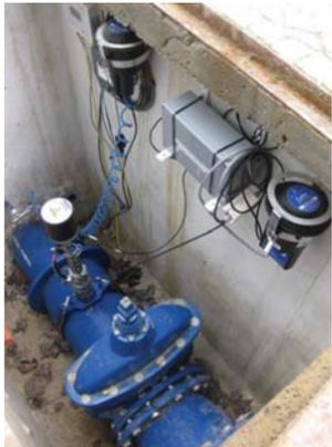
In January 2010, EPAL commenced a pilot project to monitor water quality in Lisbon's distribution network using Intellitect Water's innovative Intellisonde™ in-pipe water quality monitors. The trial sought to assess both the technology and the benefits to be gained from continuous access to water quality data between the treatment plant and the consumer.
