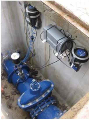
In January 2010, EPAL commenced a pilot project to monitor water quality in Lisbon's distribution network using Intellitetc Water's innovative Intellisonde™ in-pipe water quality monitors. The trial sought to assess both the technology and the benefits to be gained from continuous access to water quality data between the treatment plant and the consumer.
