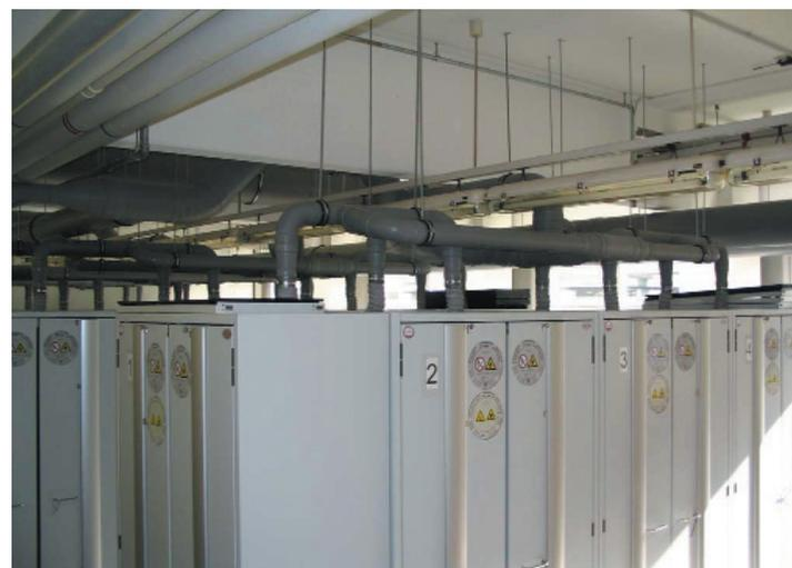
*More than 50 safety storage cabinets connected to a central ventilation system*
