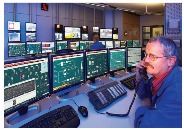
Data from emissions monitoring technology can provide valuable feedback on plant performance, enabling plant operators to optimise efficiency and operational control
